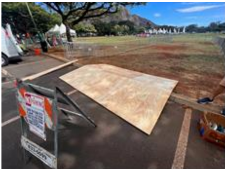
12-foot-wide Ramp in place at Kapiolani Park
